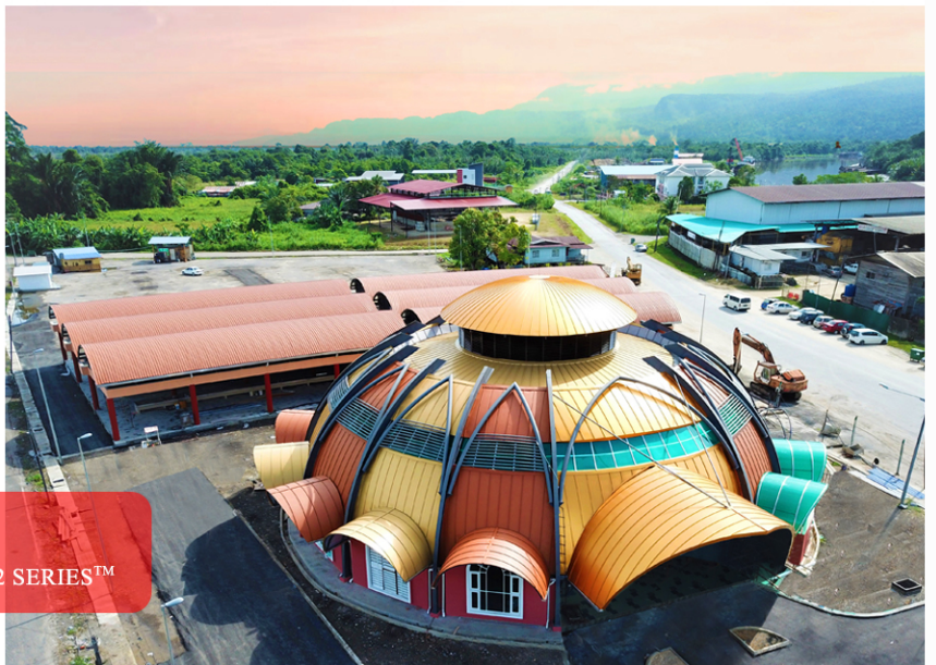
TATAU MOSQUE, TATAU IMETAL EUROSHINGLET 0.55MM TCT IN COLOURCOIL METALLIC PVF2 SERIES™
