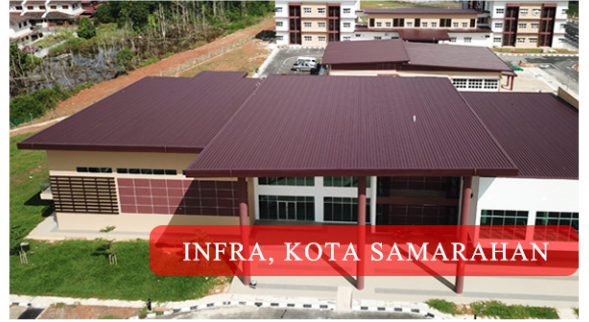
URBAN TRANSFORMATION CENTRE, KUCHING
