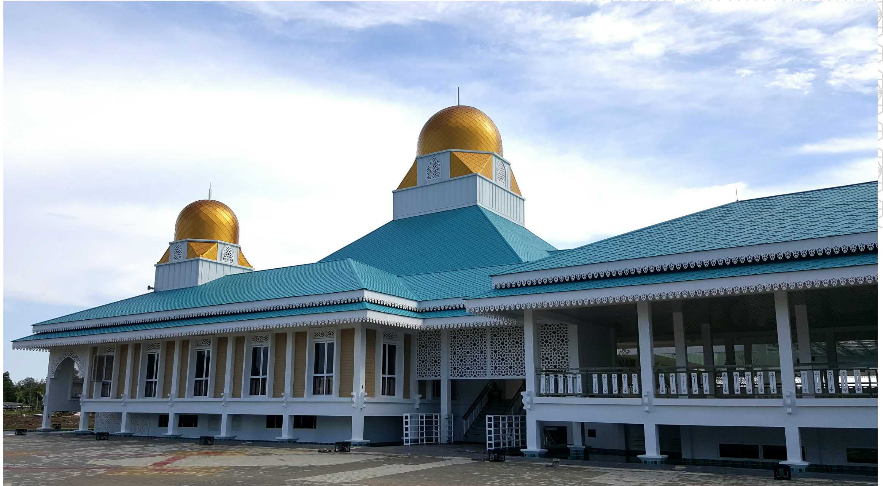
ROOFING Masjid Darul Hana | Kuching Material (Dome): Euroshingle™
