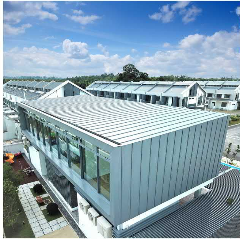
ROOFING La Promenade Clubhouse | Kota Samarahan Material: I-Seam, Elite Series™
