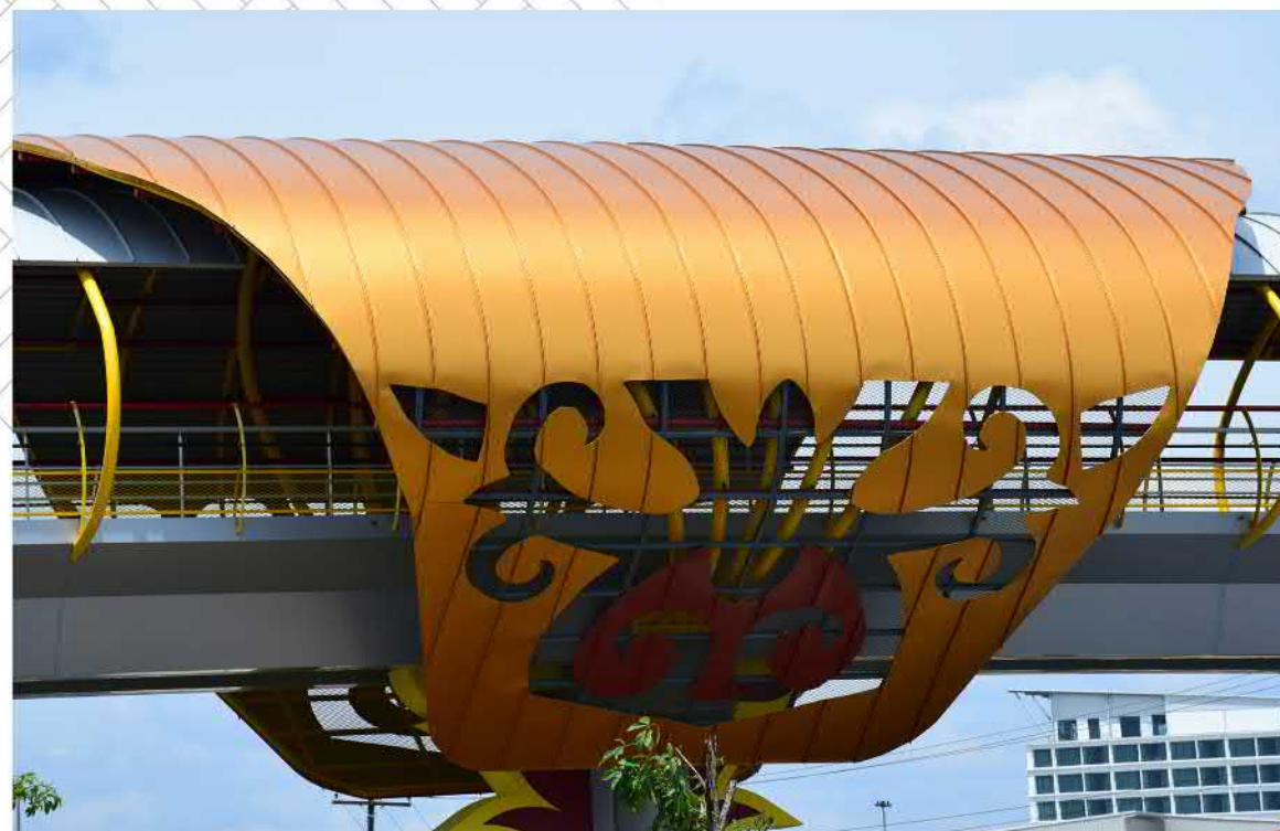
ROOFING / SCREEN & FACADES Pedestrian Bridge | Kota Samarahan Material (Roof): I-Seam Kristalmatt Series™ Material (Facade): Powder coated aluminium panels or prepainted steel sheets to be fabricated to become louvres and act as facade/screen or provide shade
