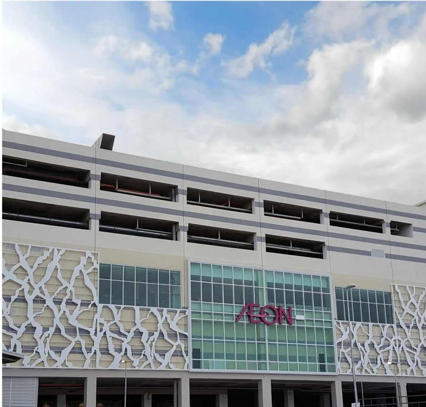
FACADE AEON Mall Kuching Central | Kuching Material (Facade): Powder coated aluminium panels or prepainted steel sheets to be fabricated to become louvres and act as facade/screen or provide shade
