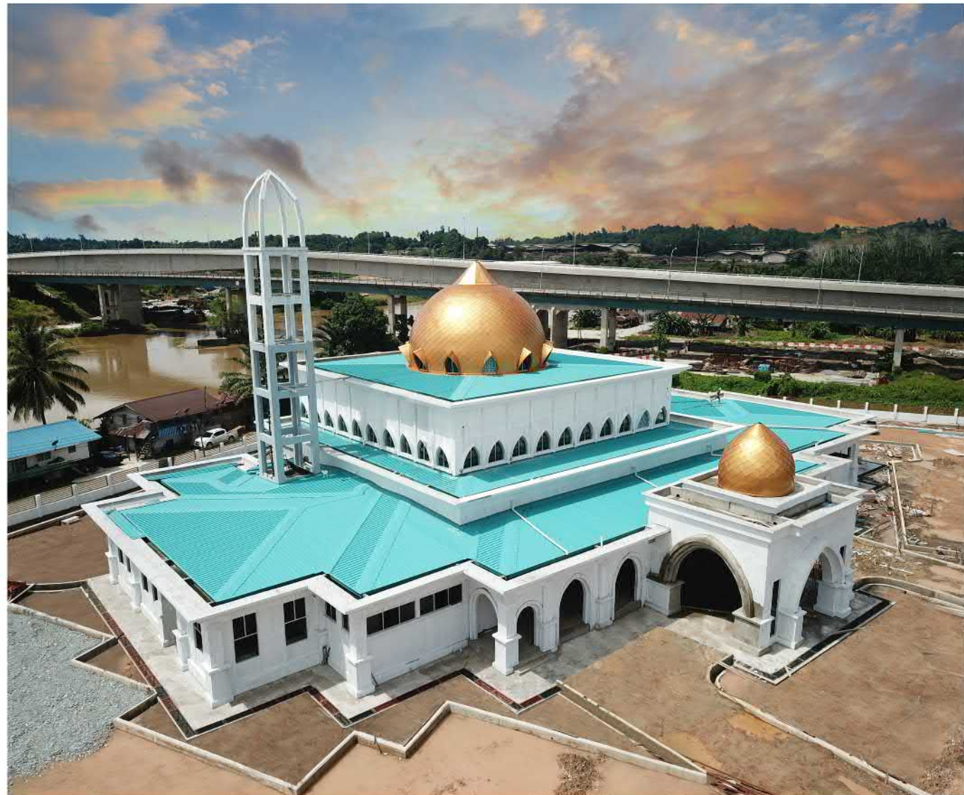
ROOFING Tatau Mosque | Tatau Material (Dome): Euroshingle, Metallic Pvf 2 Series™ Material (Roof): I-Clip, Kristalmatt Series™
